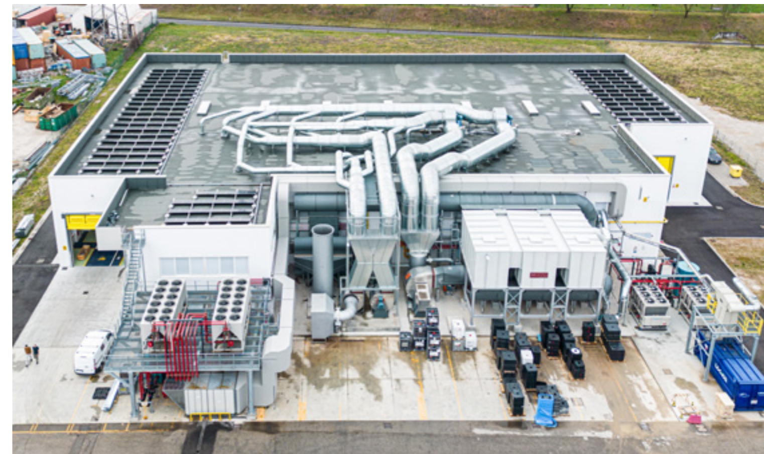
Production expansion of Line 11 in Gorizia
