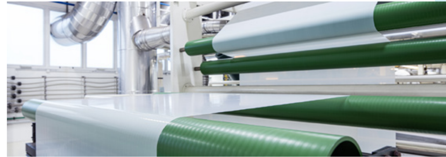
Coating production line detail
