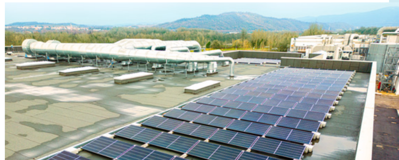
Photovoltaic panels for self-consumption of production line
